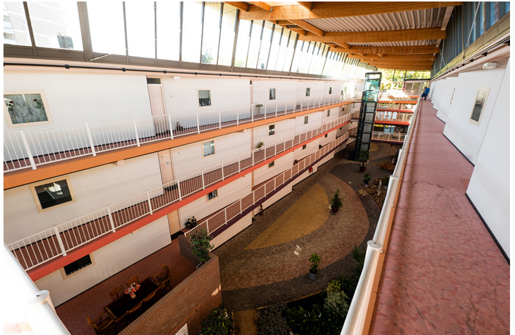
Kreilerburcht, Atrium. Photo by Jasper Mol. Maaswonen
