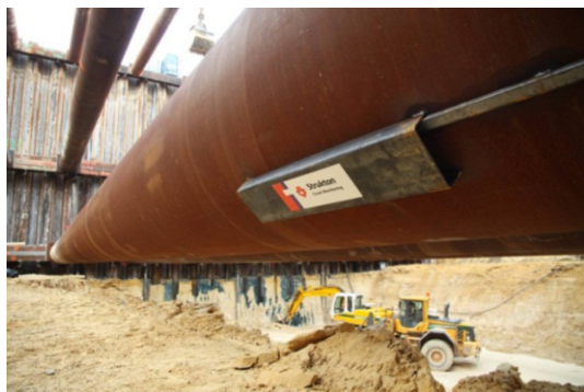
Figure 3. One out of four covered strain gages on a strut during critical excavation
