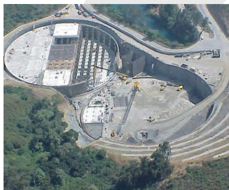
Figure 28, Hollywood Reservoir Project, Los Angeles, US
