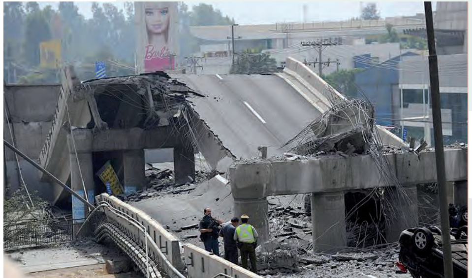
Figure 58, Earthquake Damage surface Structure, Chile (Wallis, 2010)
