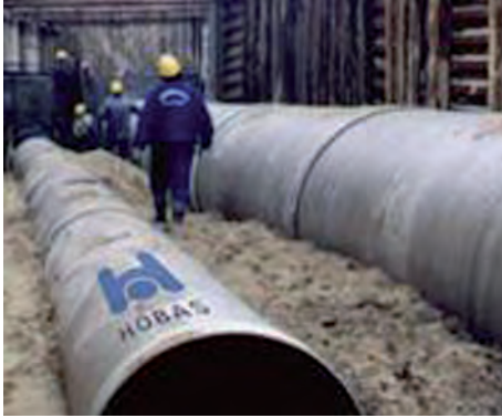
Figure 38, Pipeline in Trench Excavation
