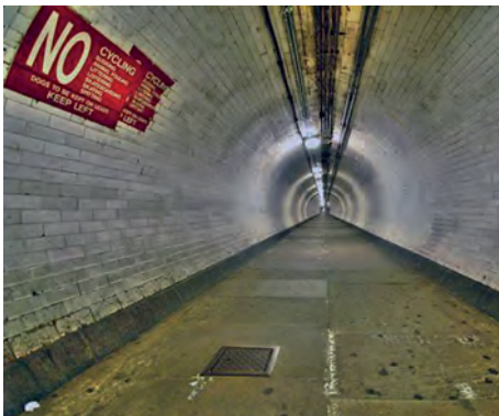
Figure 24, Greenwich Foot Tunnel, East London
