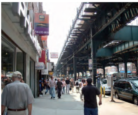
Figure 5, Aging Surface Infrastructure, New York
