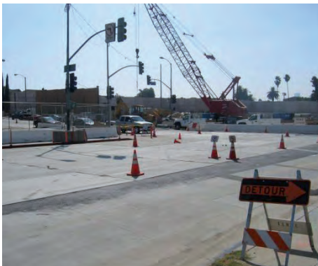
Figure 63, 'Precast concrete decking with excavation ongoing below
