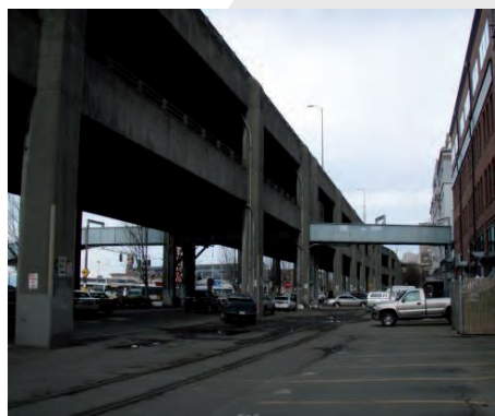
Figure 56, 'Alaskan Way Viaduct – impact on adjacent properties
