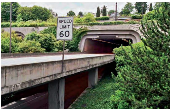
Figure 3, Mt. Baker Ridge Tunnel, Seattle, Washington, USA
