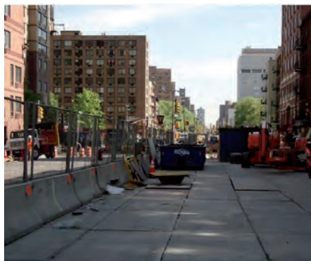
Figure 64, Cut and Cover Construction within Street, New York City
