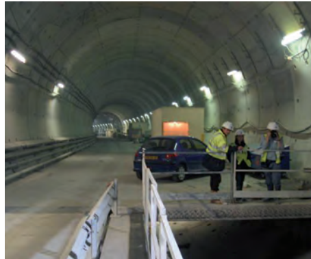
Figure 19, A86, Paris Region, Upper Deck (Photo: Cofiroute)
