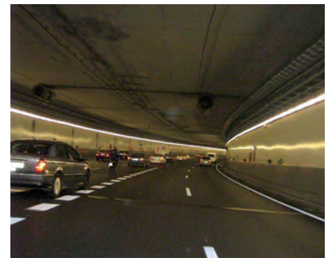
Figure 18, Road Tunnel, Calle 30, Madrid
