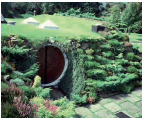
Figure 50, Earth Sheltered Housing in a National Park District, UK (architect Arthur Quarmby)
