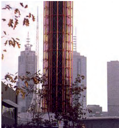
Figure 21, Melbourne City Link vent shaft
