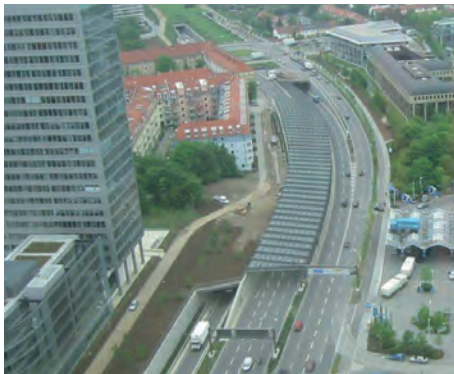
Figure 16, Ring Road Tunnel, Petuelring, Munich, Germany
