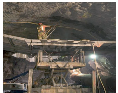
Figure 29, CSO Storage Cavern, Atlanta, Georgia, US
