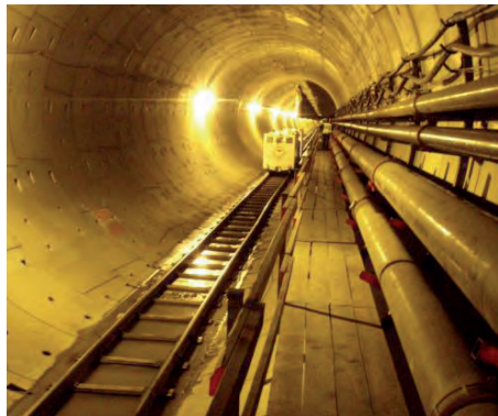
Figure 72, Modern tunneling technology
