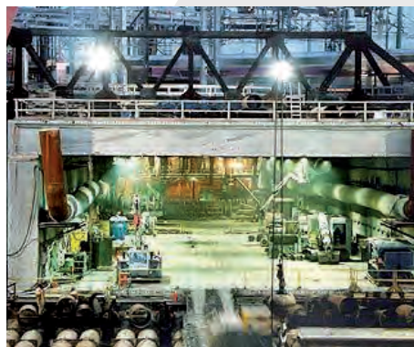
Figure 75, Ground Freezing for section under active Rail Road
