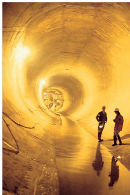
Figure 31, Tunnel Reservoir of the TARP Project, Chicago, USA
