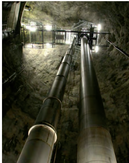
Figure 36, Underground Coal Storage, Helsinki, Finland (Photo: Jorma Vilkmán)
