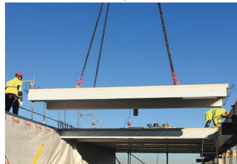
Figure 4.7: Instalment prefabricated TCC floor slab [72]
