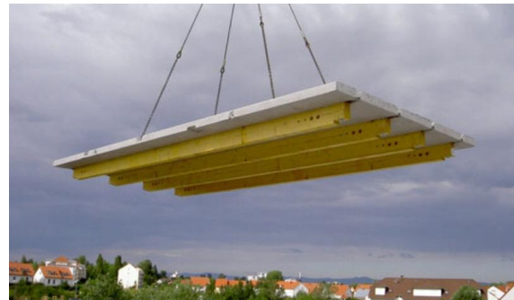
Figure 4.2: Timber-Concrete Composite rib floor [67]
