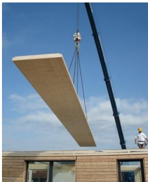
Figure 2.28: CLT floor [5]
