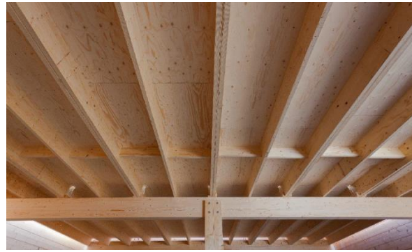
Figure 2.26: Wooden rib floor [16]
