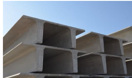
Figure 2.15: TT slab floor [7]
