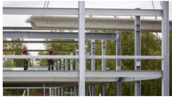
Figure 2.11: Instalment TT-slabs parking garage ASML [13]
