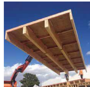
Figure 4.3: Prefabricated LVL floor unit [1]
