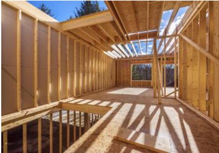
Figure 2.7: Timber frame construction [37]
