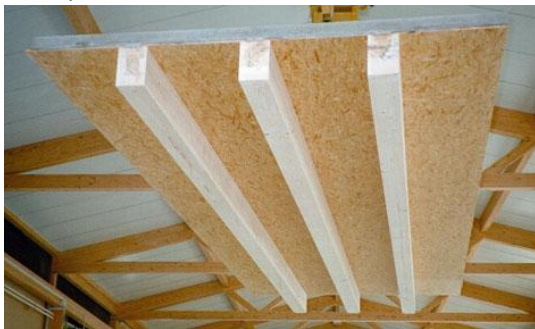
Figure 4.6: Prefabricated TCC floor slab [71]
