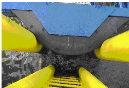
Figure 5-7: A top view of a fender interacting with the wind turbine’s boat landing [71]
