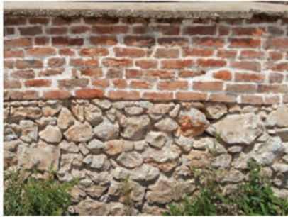
MIX WALL (DRY STONE & RED BRICK)
