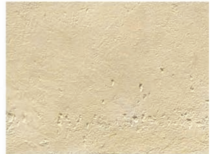
PLASTERED WALL (PAINTED)
