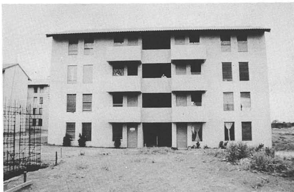
One of the first four-storey blocks
