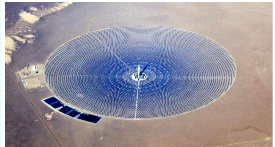
Figure C16: Crescent Dunes Solar Energy Project plant (Boretti A., 2020).
