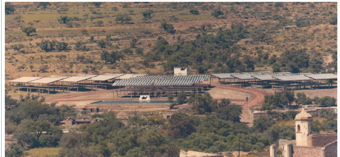
Figure C9: SOFRETES solar-powered water pumping plant in Guanajuato, Mexico (Pytlinski, 1978).
