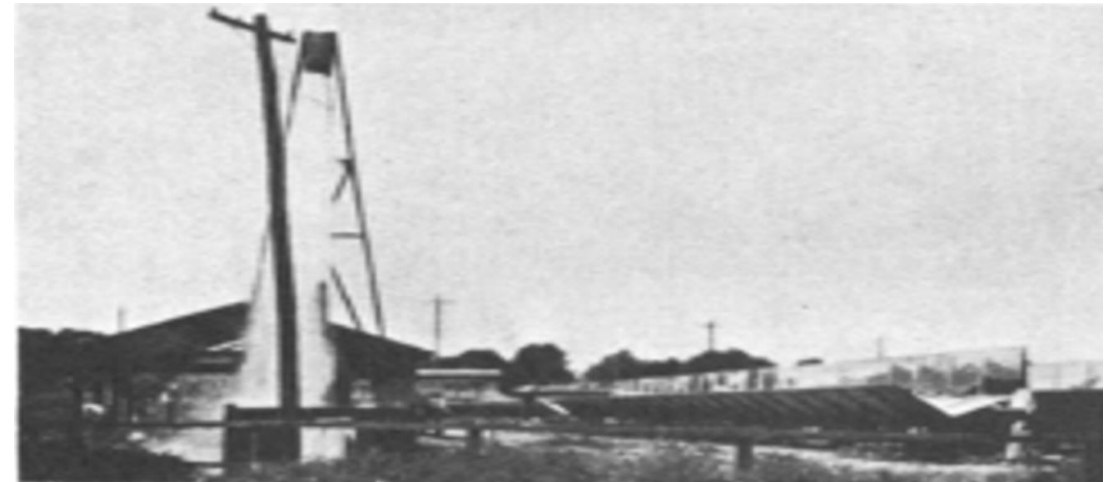
Figure C3: Shuman's solar-powered irrigation installation. (Pytlinski, 1978)
