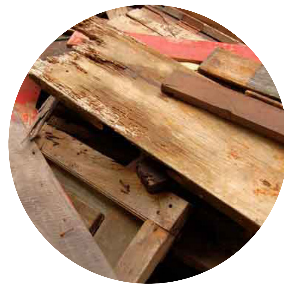
Beams and planks
