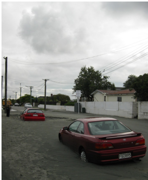
Figure 2.2: Soil Liquefaction - Christchurch Earthquake 2011, Source: Timothy Musson
