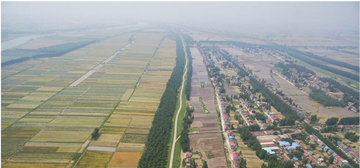
Fig.2.6. Unbalanced spatial distribution in Jing River Flood Storage Area in Jiangnan Plain
