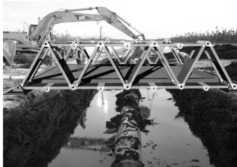
Figure 7.6 | Application of DeMoLi in construction site
