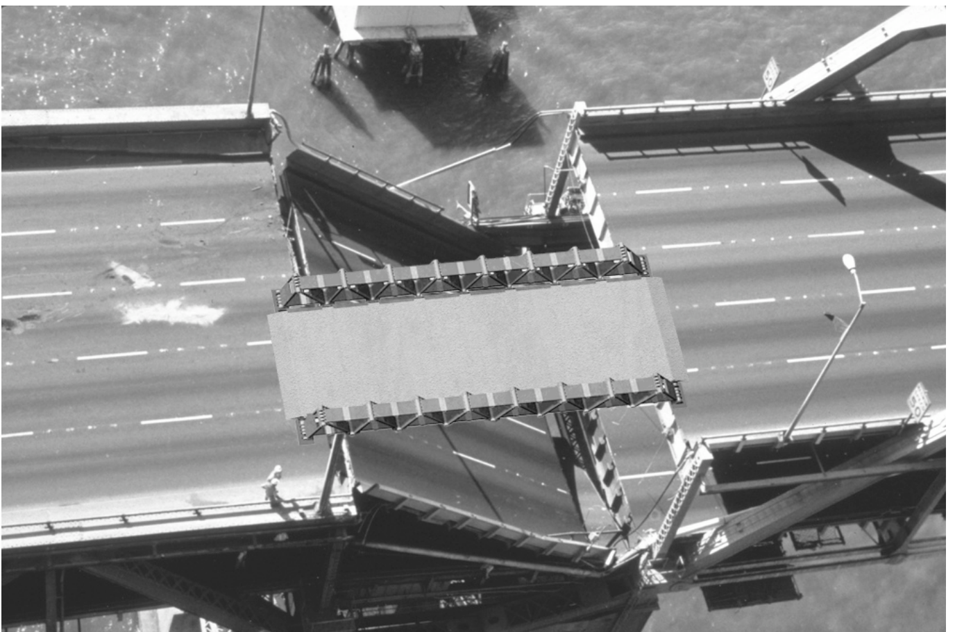
Figure 7.3b | Application of DeMoLi12 in Bay Bridge, in Northern California
