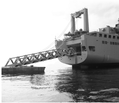
Figure 7.4 | Application of DeMoLi12 in maritime Roll-On Roll-Off (RORO) ramp
