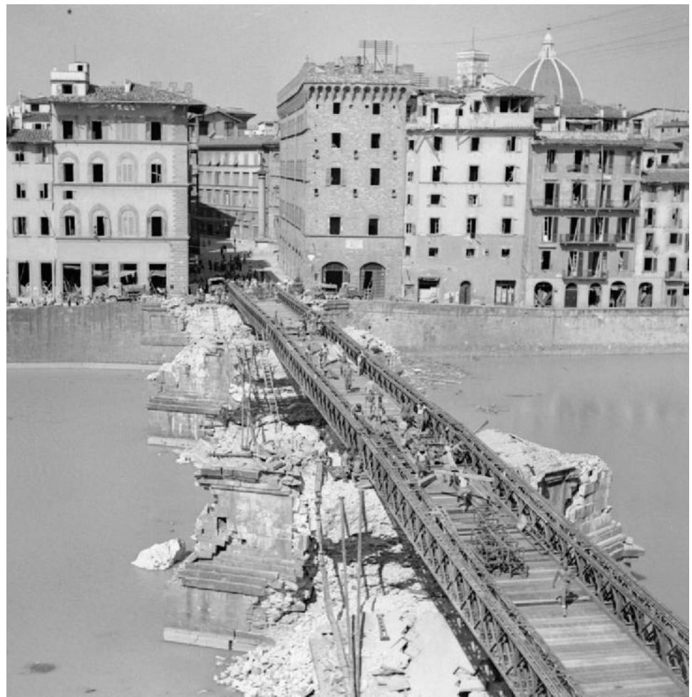
Figure 1.4 | Bailey Bridge (or Heavy Girder Bridge)
