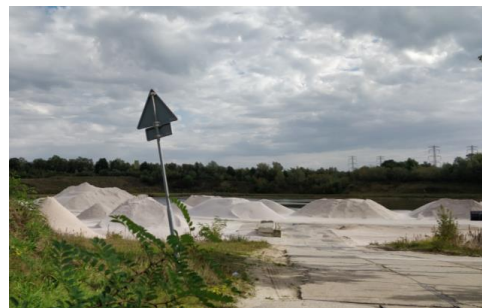
Water pollution Generally contains heavy metals or additives used in mining industry. Rising mine water can lead to an increase in groundwater level in the overburden. Due to this groundwater is at risk.
