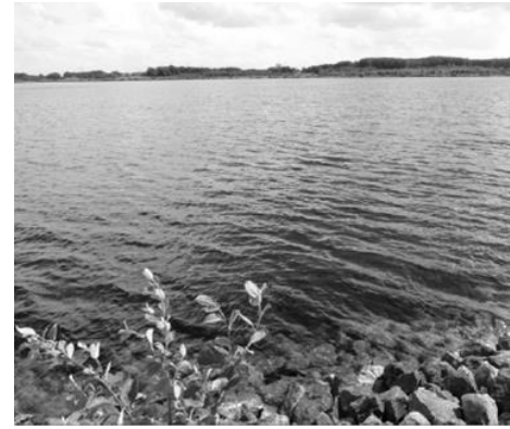
Drinking water extraction
