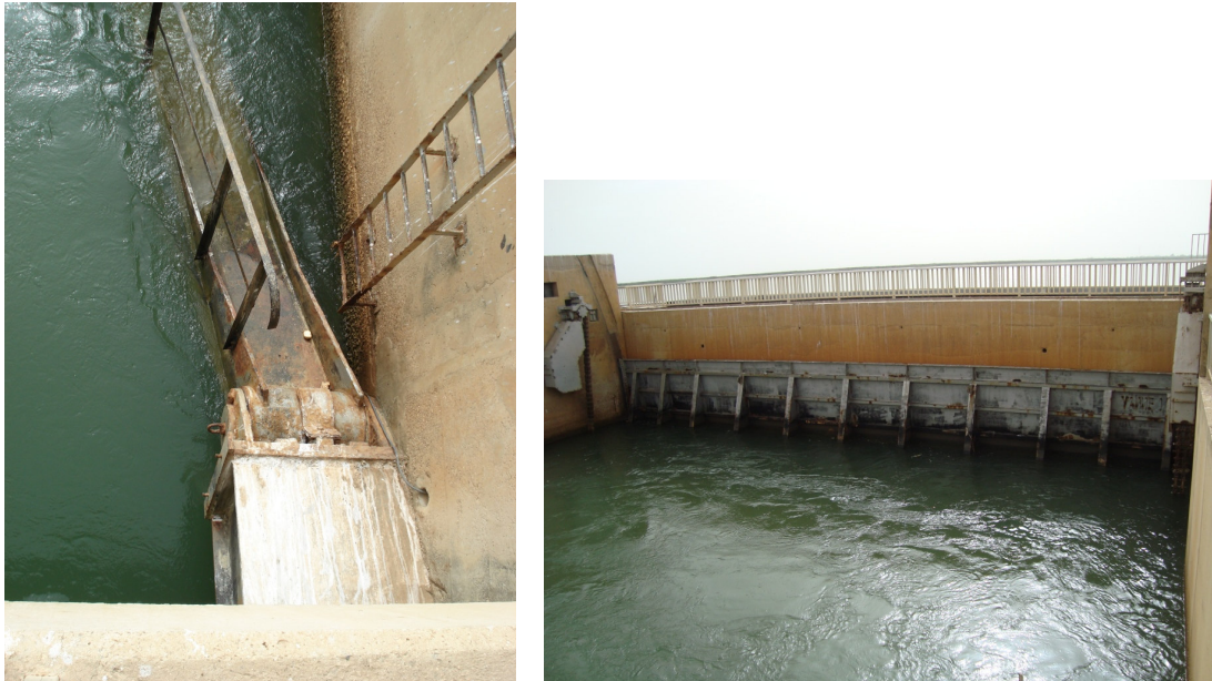
Figure 4-10: Rotation point for dam gate (left) and the gate itself (right). (Source: personal picture)
