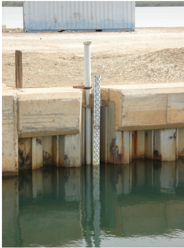
Figure 4-15: Gauge at the Diama dam. (Source: personal picture)
