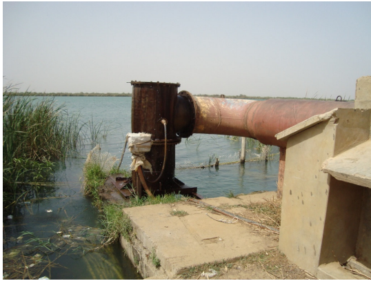
Figure 4-6: Water extraction structure for irrigation. (Source: personal picture)
