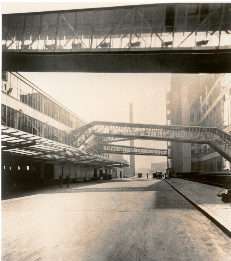
Figure 5: Van Nelle factory, bridges connecting the three volumes.
