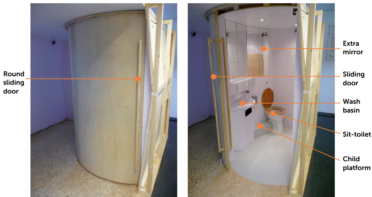
Figure 7.1a exterior and 7.1b interior of mock-up 1: family sit-toilet module
