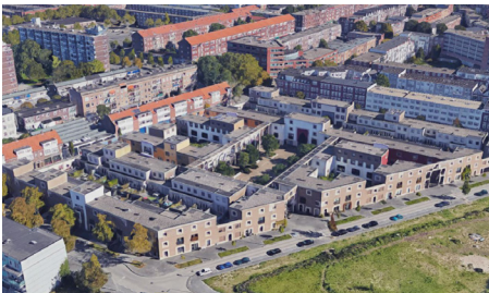
AERIAL VIEW LE MEDI FROM WEST
