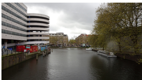
SINGELGRACHT AND ADJACENT PARKING GARAGE
