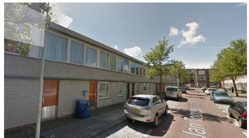
NORTHERN FACADE PUNT
