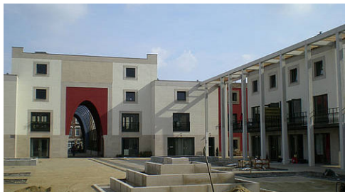
Interior Central Square (Afritecture)
