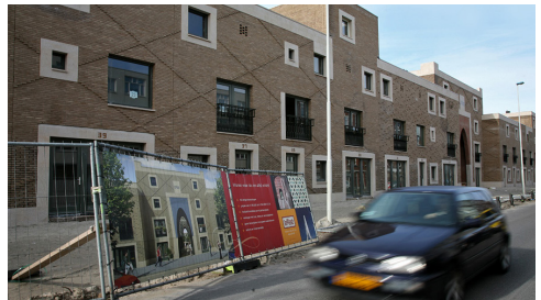
Exterior facade (Afritecture)
