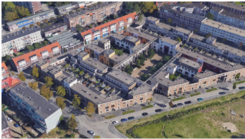
AERIAL VIEW LE MEDI FROM WEST
