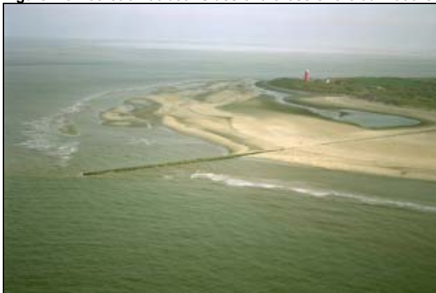
Figure 4-5 Accretion at both sides of a cross-shore dam at the island of Texel (Wadden Sea)
