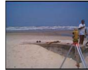
Total station / distance meter + survey rod
