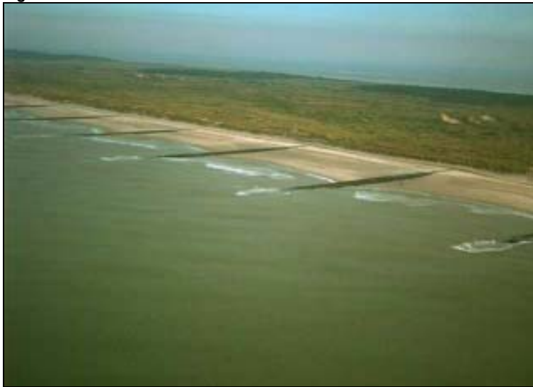
Figure 4-3 Groins at the Wadden island Vlieland in the Netherlands
