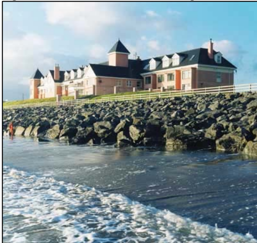
Figure 4-6 Armoured section at Donegal
