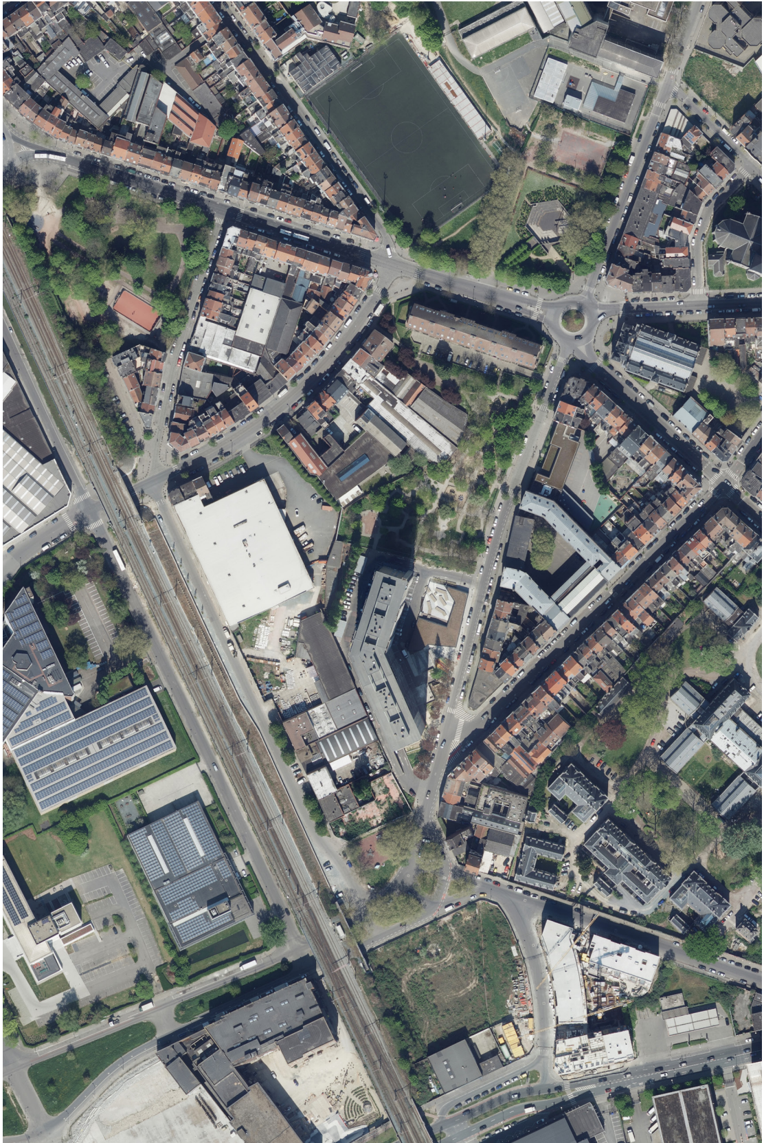
Fig. 54. Aerial picture from the 2020. Source: www.bruciel.brussels/#
