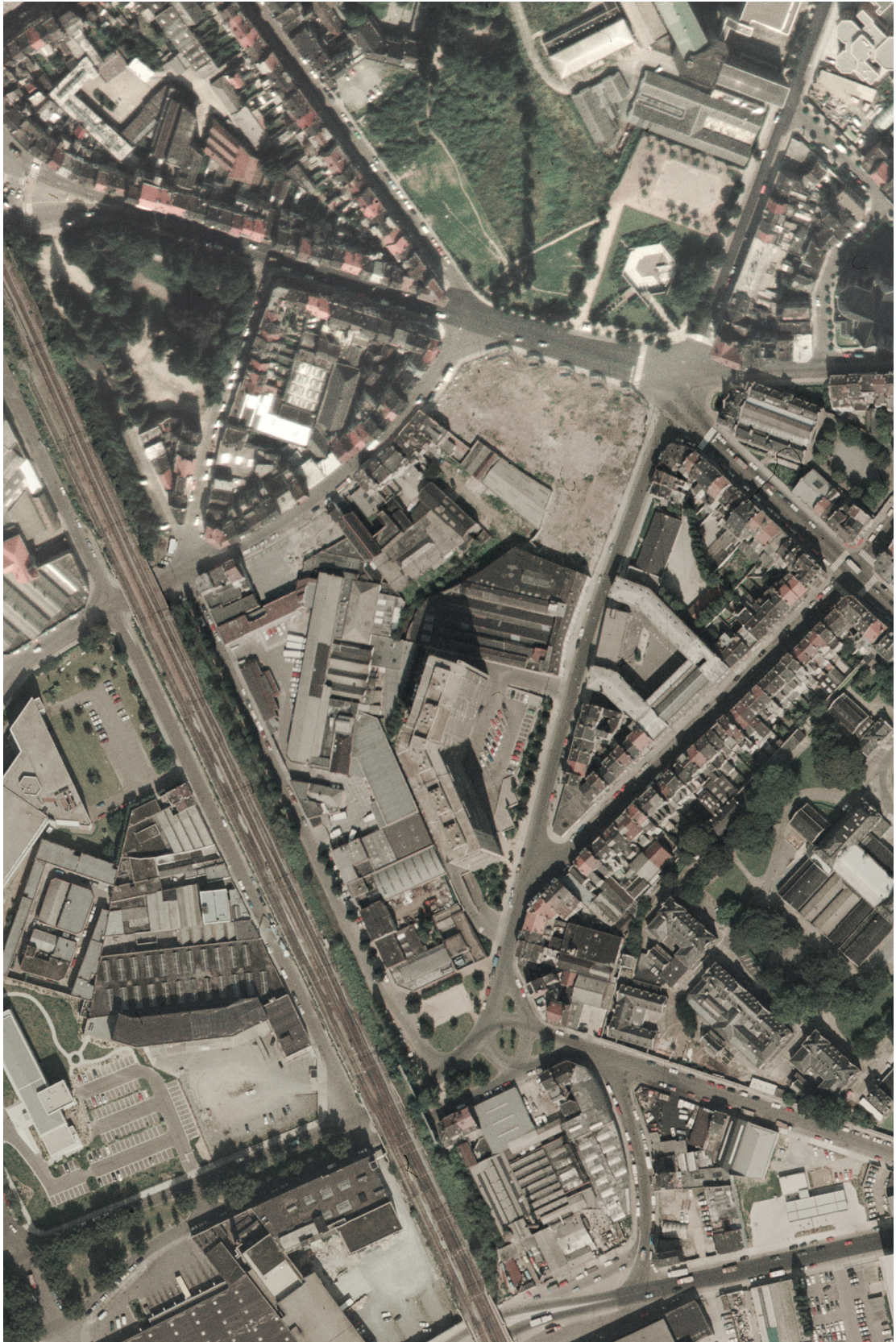
Fig. 51. Aerial picture from the 1987. Source: www.bruciel.brussels/#
