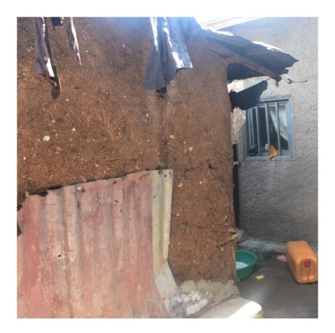
A traditional way of wall construction used throughout Ethiopia is Chika: a load-bearing wall with eucalyptus wood as frame structure and mud as infill. Some people opt to also add a layer of cement plaster on the mud surface as a water barrier. This construction method utilises local materials and is part of the vernacular architecture lineage. The downside is that this method cannot sustain more than 2 floors and is susceptible to erosion.
