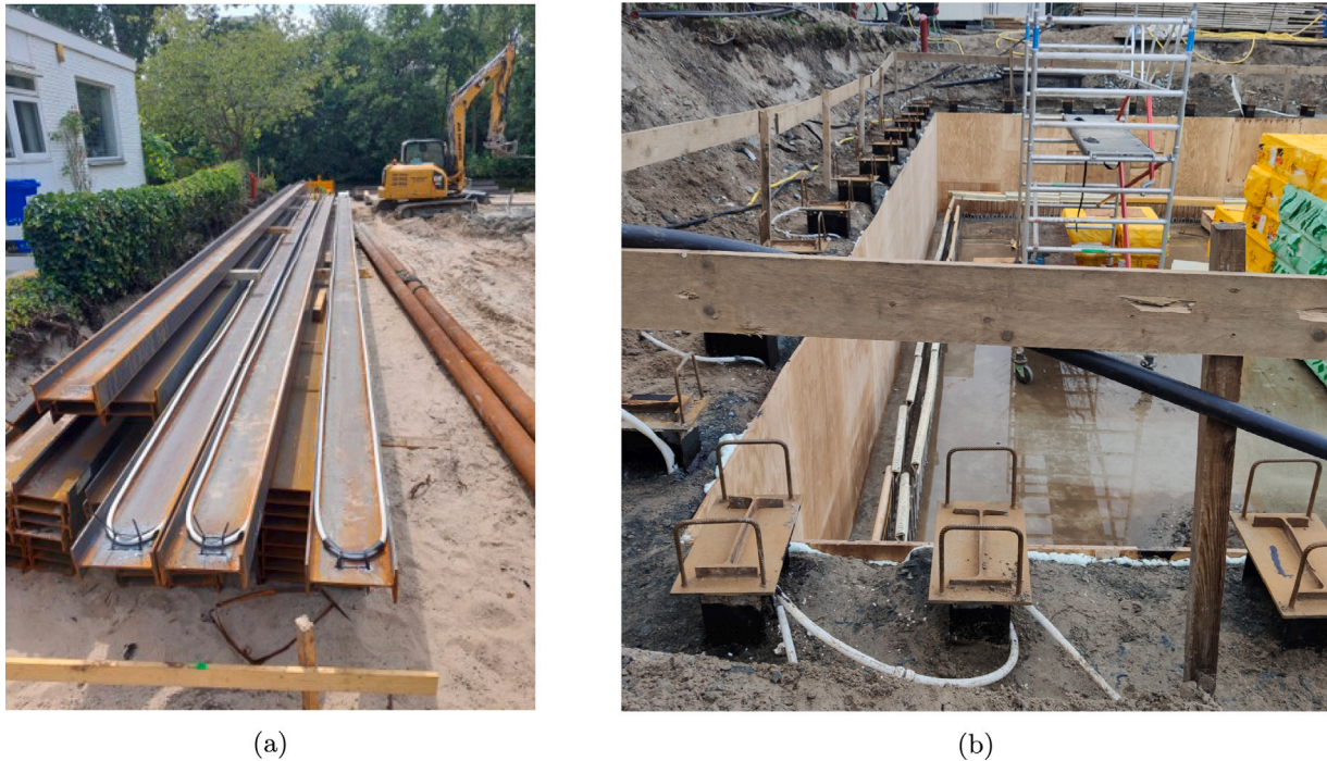
Fig. 2. CSM full-scale test installed in Amstelveen (NL): (a) heat exchanger pipes on the steel IPE300 profiles, and (b) CSM energy wall full scale test.
