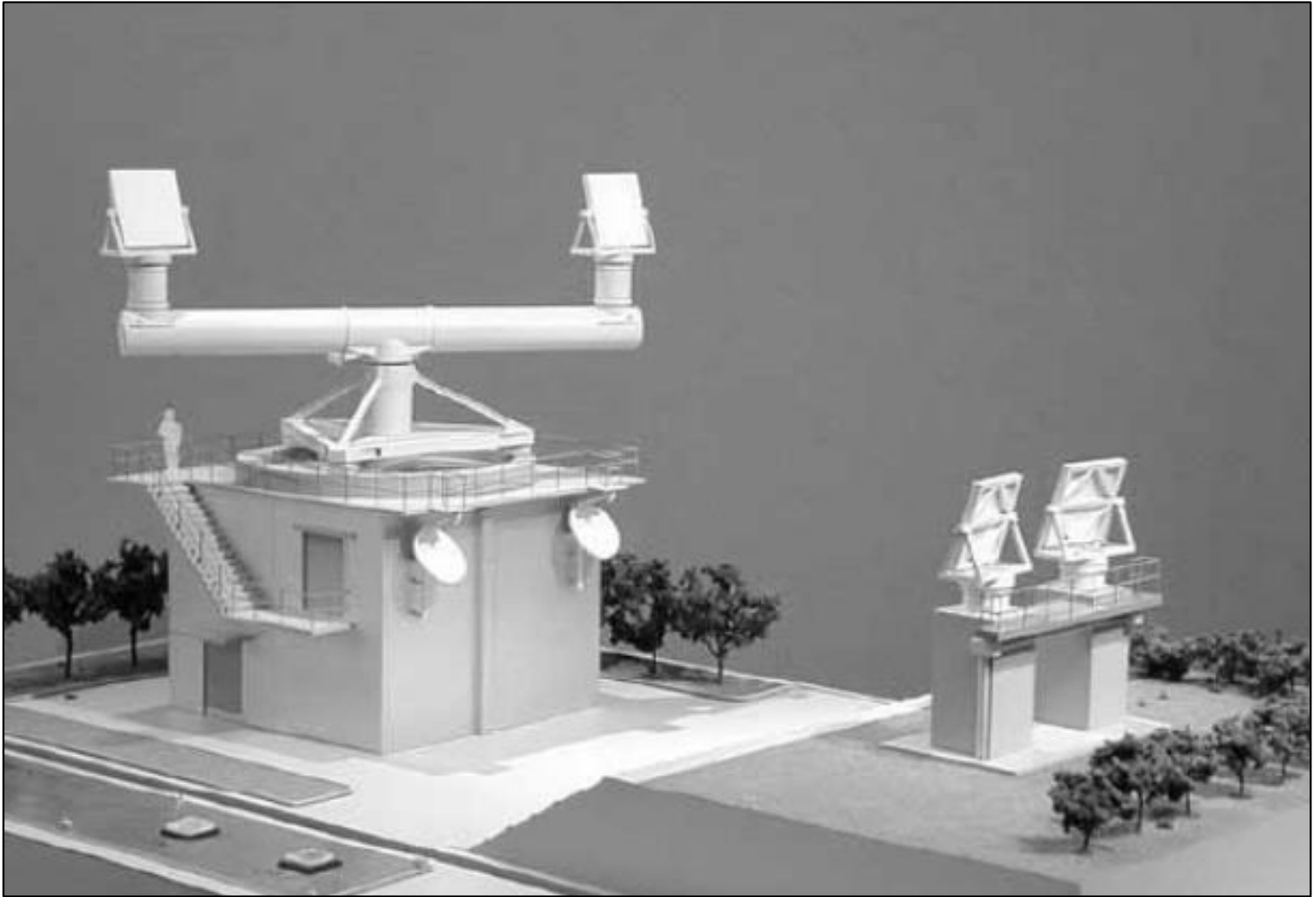
Figure 7: scale model of a rotary reflecting phase interferometry ground station, note human for scale [25]
