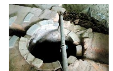
Fig. 3-3-17(up) Seepage well in ancient Canton Source: Liu (2015)
