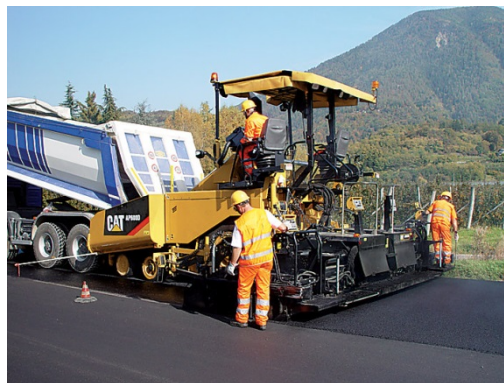
Figure 5.2 Asphalt paver for asphalt mixture distribution [58]
