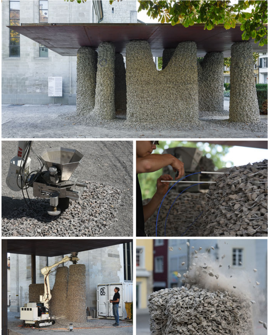
Fig. 9.1 (i) The Rock Print Pavilion is a full-scale robotically jammed structure composed of gravel aggregates and twine. The enabling technologies facilitating the on-site adaptive construction process include a custom robotic end-effector (ii) for extruding twine, depositing aggregates, and compacting layers, a structural health monitoring approach for the movement of the structure and the roof over time (iii), and mobility and localisation of the IF enabling the production of a larger structure on uneven ground (iv). The structure can be easily deconstructed with no material downgrading by removing the twine (v). (© Georg Aerni)
