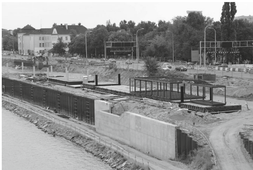
Fig. 8 Construction process on the amphibious pavilions in Warsaw in June 2017. Dolphin piles, concrete foundations, and steel pontoons are visible (image taken by author)
