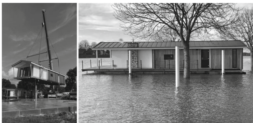
Fig. 5 Chalets with aluminium foundation during construction and afloat during floods (source Resort Marina Oolderhuuske)
