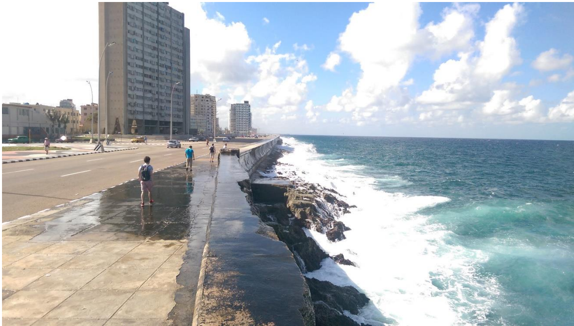
Figure 6: View of section 2 as seen from the seawall
