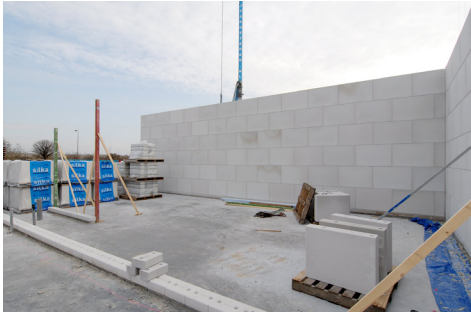
Artificial sand-lime stone walls used for the stability disc walls as a sustainable wall type Calduran
