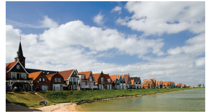
Figure 19: Volendam dike needs strengthening
