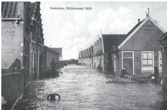
Figure 8: Flooding in 1916 (Hart)
