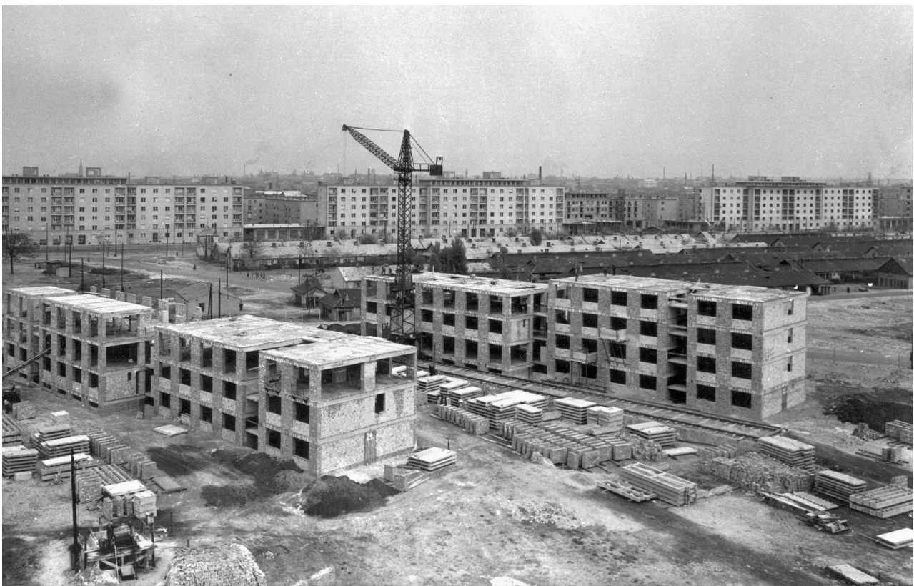
Fig.3. József Attila Estate Pöttyös street, Hungary The first stage of the mass housing plan began. The prefabricated panels are visible in the picture. (Ferencvárosi Helytörténeti Gyűjtemény, 1959)
