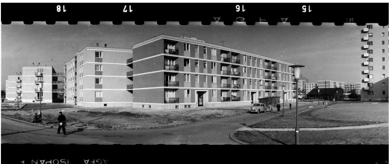
Fig. 7, First buildings Budapest, Hungary, József Attila Housing Estate just after completion, Dési Huber Street on the left. Unfinished landscape and infrastructure are visible, the roads are still covered with dirt, grass is not yet grown. (Gábor Viktor, 1961)
