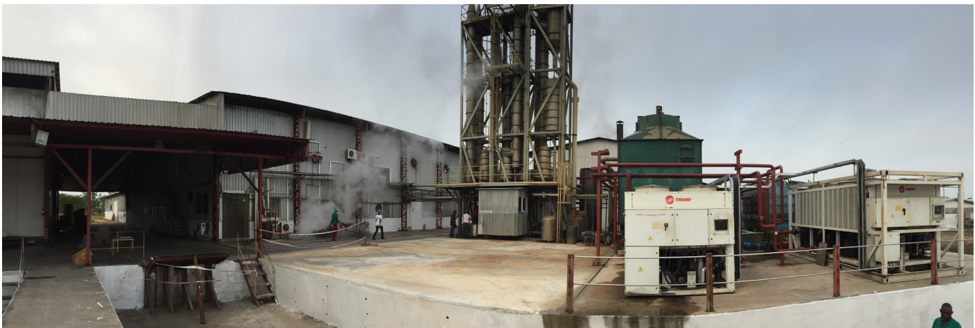
Figure 51. Overview of the facility. Including a “trench” for a truck, so that the mouth of the truck is at the same level as the factory floor. At some customers nearby juice producers, drum need to be “dropped” out of the truck.
