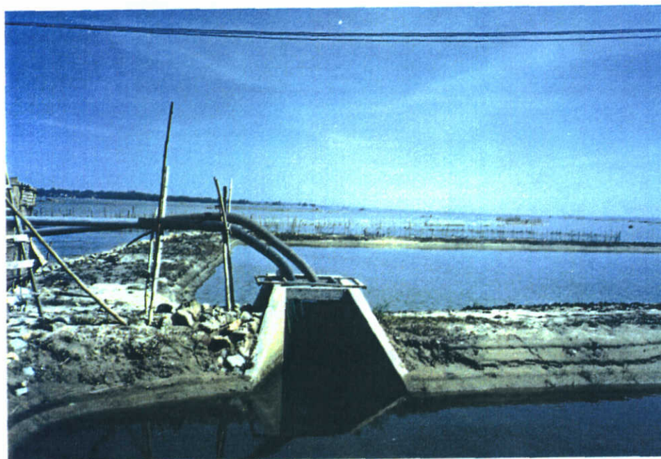
Flow control facilities in shrimp ponds
