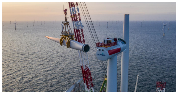
Figure 1.1: Traditional installation method: assembly at sea (source: (OffshoreWIND.biz, 2025))
