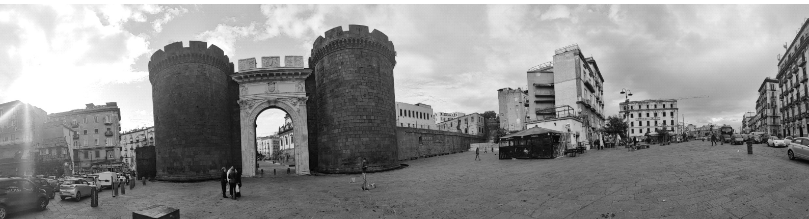
Fig. 92 Current Situation at Porta Capuana looking to the West
