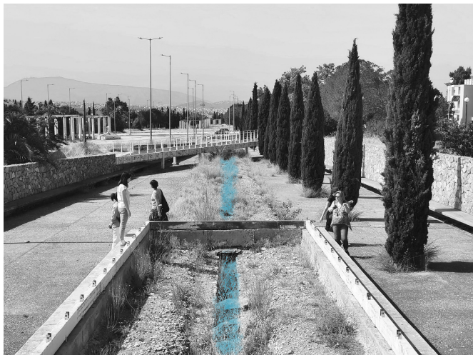
Fig. 65 Intervention point along the Hadrian Aqueduct in Chalandri (Source: Cultural HIDRANT FB page)
