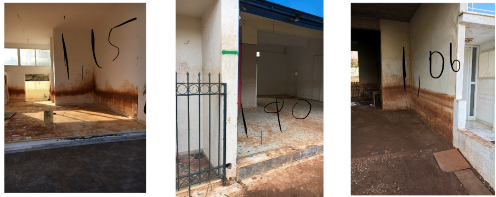
Figure 5. Indicative observation points in Mandra town (inside the buildings): the observed maximum depths are 1.15 m (left), 1.90 m (middle), 1.06 m (right).
