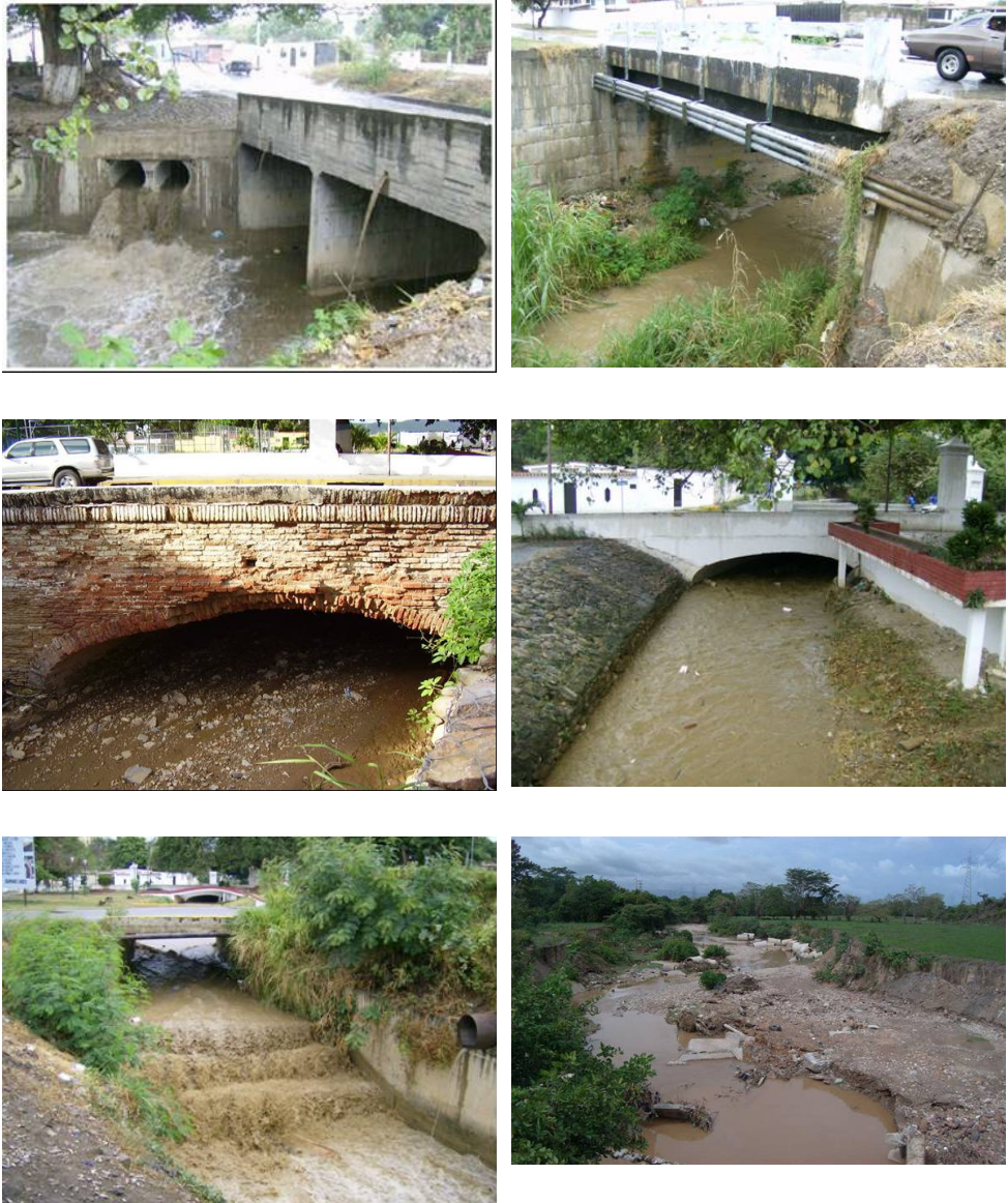
Figure 7.6: Control structures and channel cover in Tabure River
