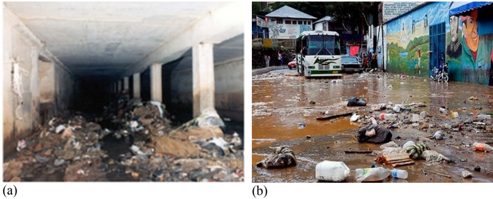
Figure 1.3: (a) Garbage accumulated in a drainage conduit in Belo Horizonte-Brazil (b) litter after a flooding event in Caracas-Venezuela
