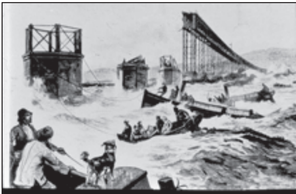
Bridge over the Firth of Tay.
