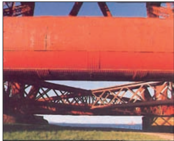
Firth of Forth Bridge
