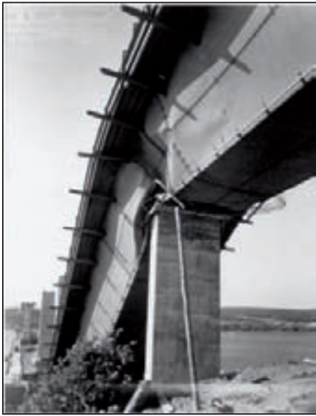
Collapse Milford Haven Bridge (Foto Inst. Struct. Eng.)
