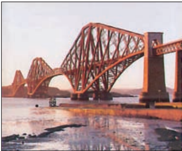
Firth of Forth Bridge
