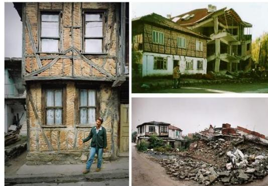
Figure 23: Left: an example of a Hımiş building suffering only plaster cracks after the 1999 earthquake, Top right: View of Hımiş house next to a RC building after the 1999 Düzce earthquake. Bottom right: View in Adapazari with Hımiş house on left beside several blocks of pancake collapsed RC buildings
