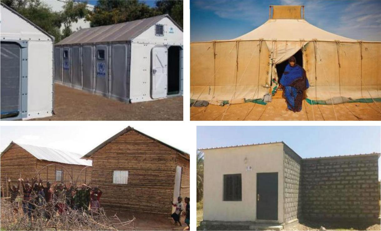
Figure 20: Four types of shelter - Right top: RHU unit global shelter, Left top: Tuareg tent in Sahrawi (emergency shelter), Right bottom: Compact bamboo shelter Ethiopia (Transitional shelter) and Left bottom: Shelter in Iraq (durable shelter)
