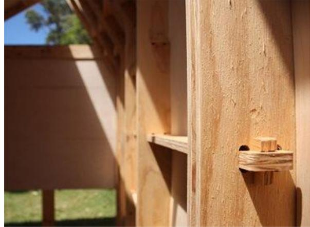
Figure 66: A wedged mortise and tenon joint
