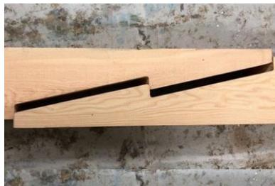
Figure 43: Scarf joint
