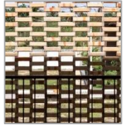
Perforated red bricks
