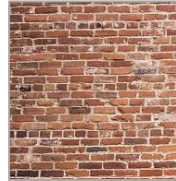
Wall, ceiling Red bricks
