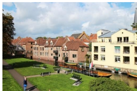
Façade A (Before renovation)
