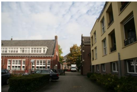
Façade A (Before renovation)
