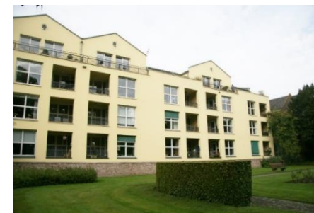
Façade D (Before renovation)
