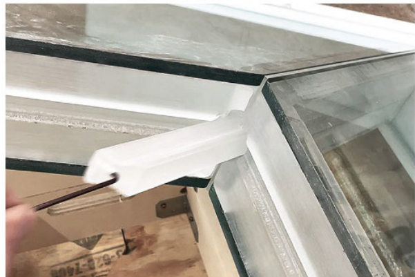
Figure 60: A locking strip is inserted into the channels of two neighbouring HGUs
