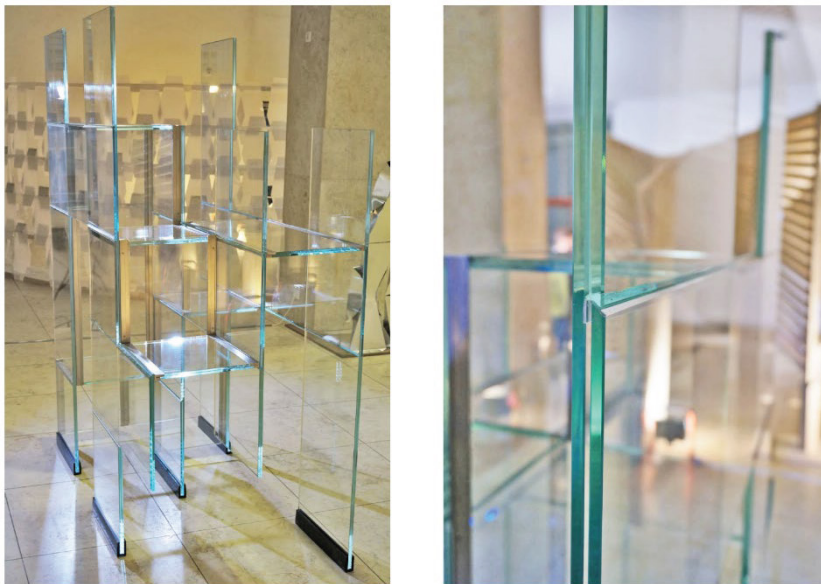
Figure 49: Exhibition of the prototype at TU Munich, detail of the glass joining method. Source: Eversmann, P., & Ihde, A. (2018). Laminated Glass Connection Details: Towards Homogeneous Material Joints in Glass .
