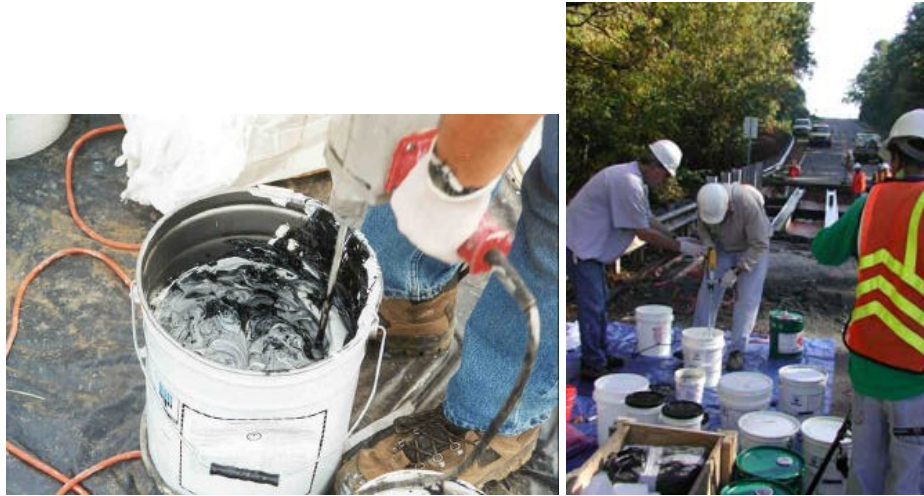
Figure 2-70 Mixing of Adhesives (Winkelman, 2002), (Craig & Sweet, 2005)
