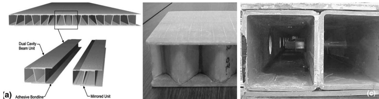
Figure 2-20 Deck panels through various joining techniques. (a) Bonded pultrusion shapes (b) Bonded sandwich (c) Bonding with fastening (Zhou & Keller, 2005)
