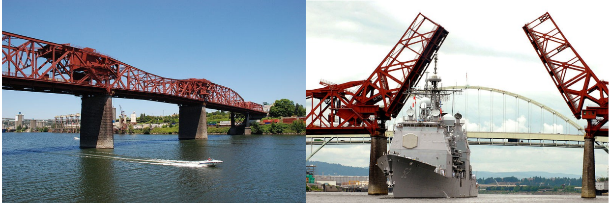
Figure 2-82 View of the Broadway Bridge (Wikipedia, 2012)
