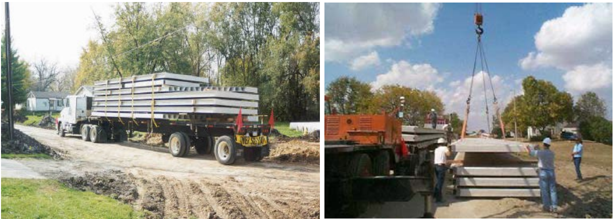
Figure 2-69 Panel Delivery by Tractor-Trailer (Winkelman, 2002) (Craing & Sweet, 2005)
