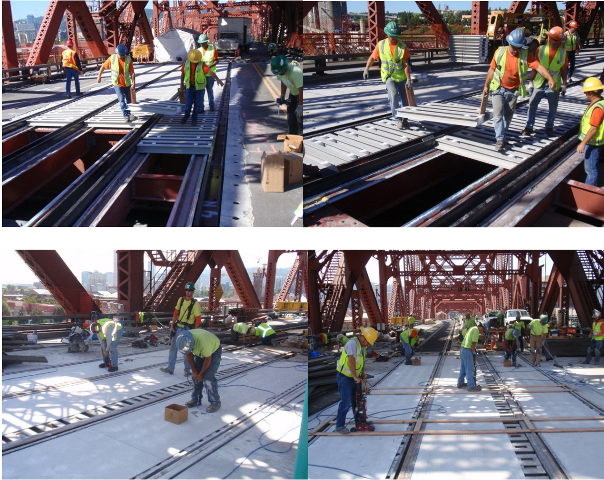
Figure 2-87 Installation of bottom sections and top sheets (ZellComp, sd)
