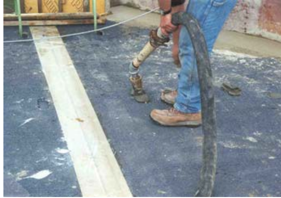
Figure 2-73 Installation of Grout (Craing & Sweet, 2005)
