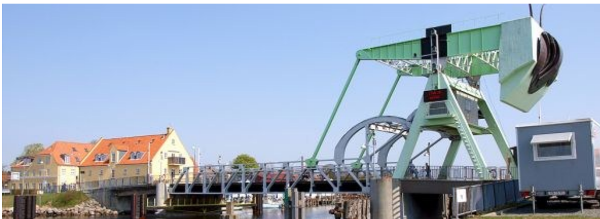
Figure 2-79 Side view of the Grasshopper Bridge, Denmark (Fiberline)
