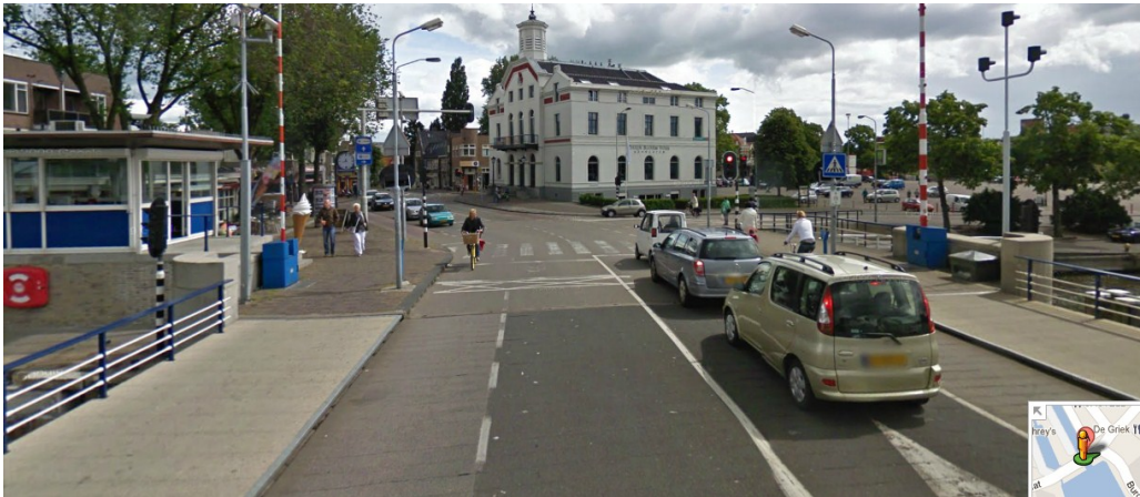
Figure 3-3 Street view of Wilhelmina Bridge
