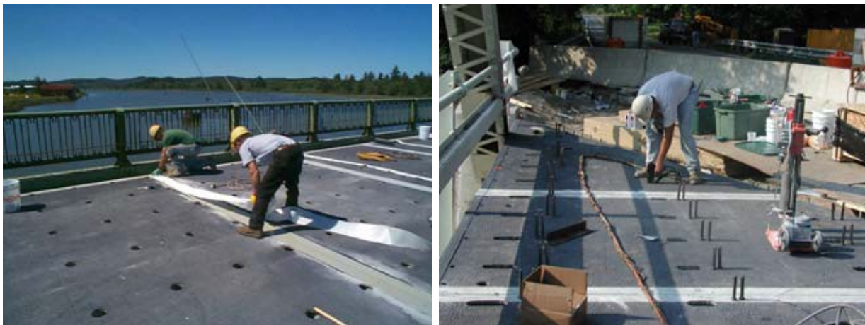
Figure 2-72 Applying Field Splice Joints (left) and Shear Studs (Right) (Craig & Sweet, 2005)
