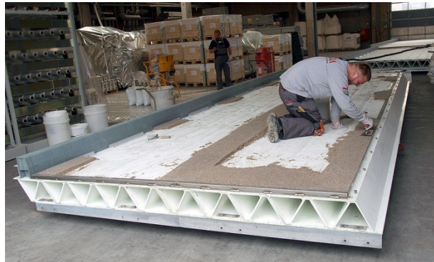
Figure 2-80 Preparation for work (Fiberline)
