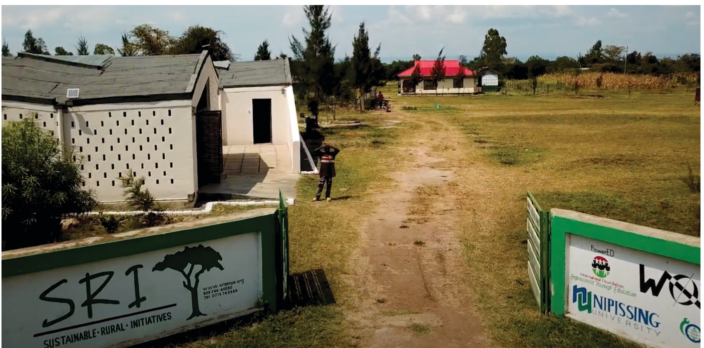
Figure 21: SRI’s community centre as viewed from the road
