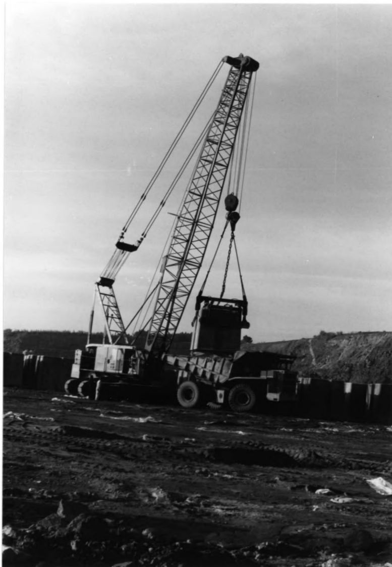
BLOCK FABRICATION SITE.(PICTURE 5)
