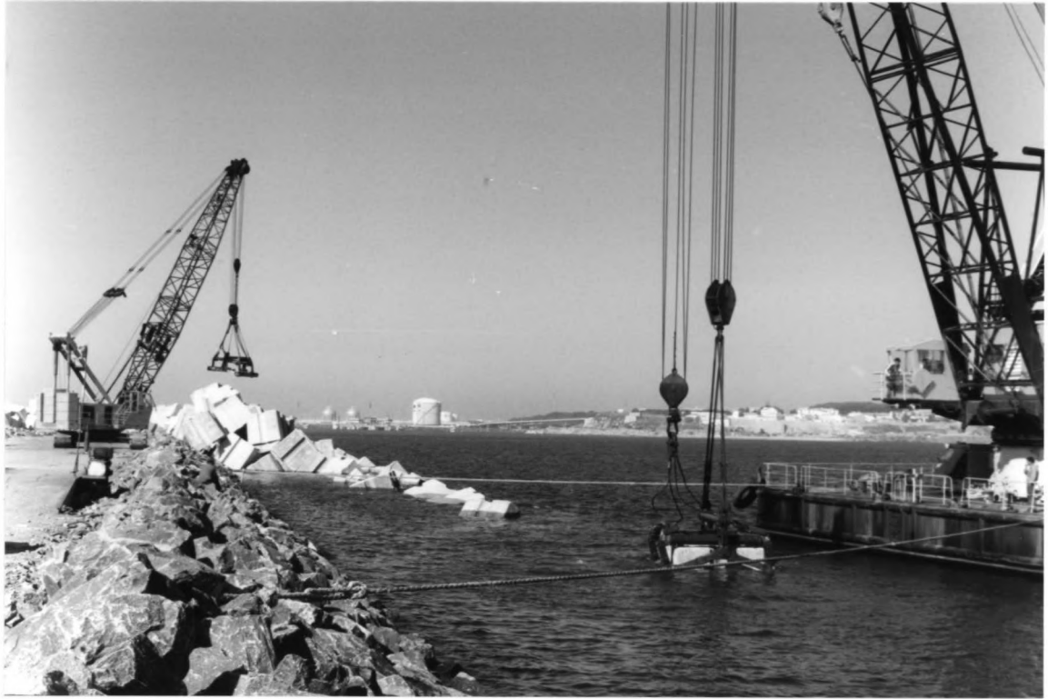
INSIDE SLOPE OF BREAKWATER ( PICTURE 6 )
