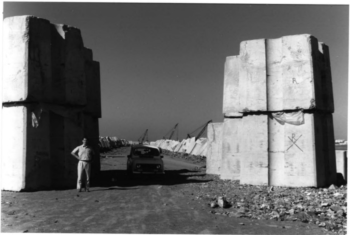
BLOCKS USED AS FORMWORK FOR CAPWALL ( PICTURE 7 )
