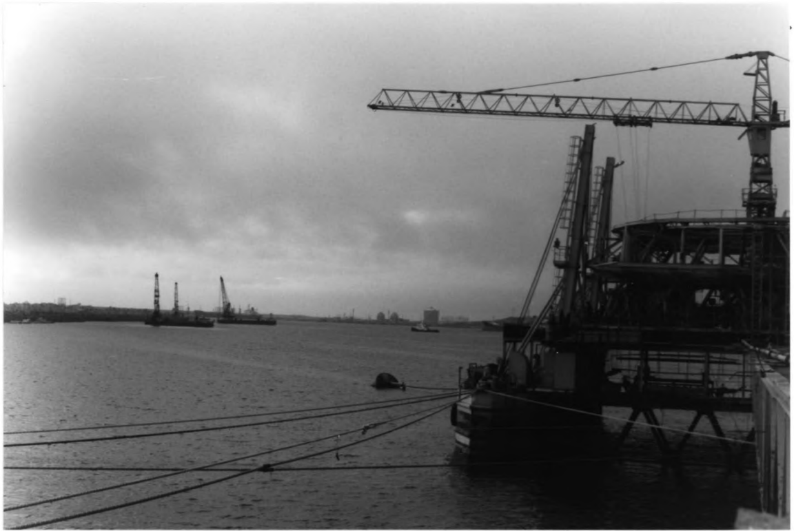
CAISSON BUILDING PONTOON (PICTURE 8)
