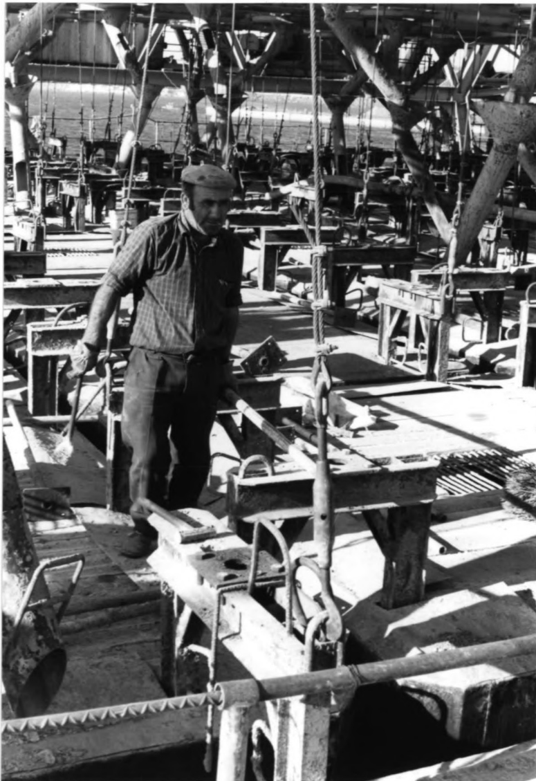
DETAIL SLIDING-FORMWORK (PICTURE 9)
