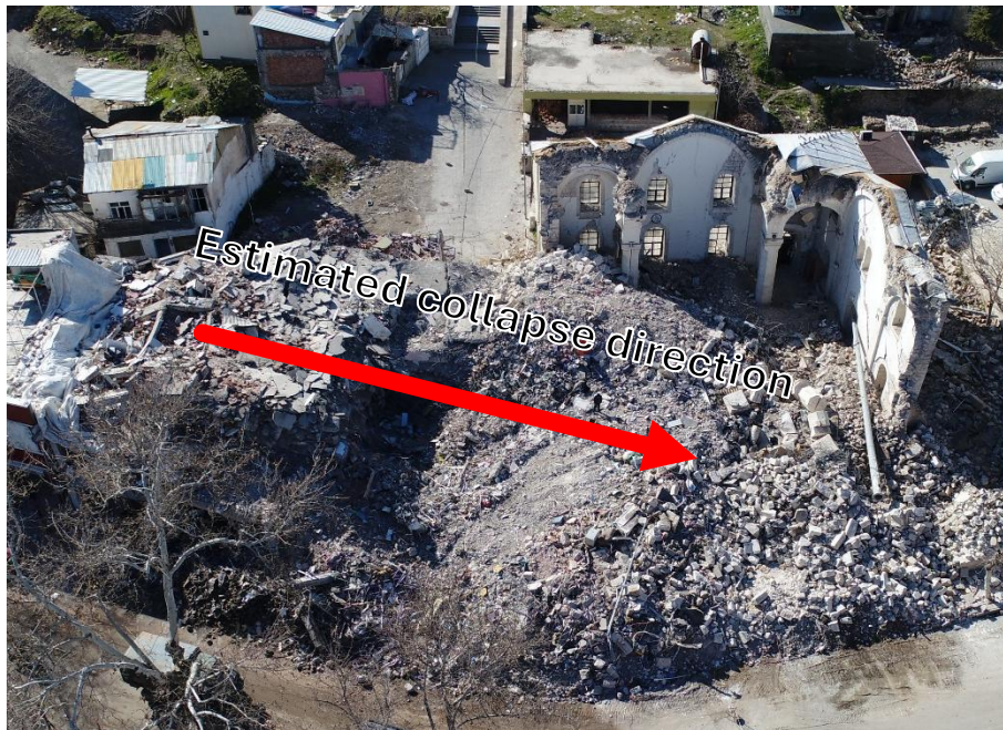
Figure 7-4 Photographic evidence indicating collapse direction toward the mosque.
