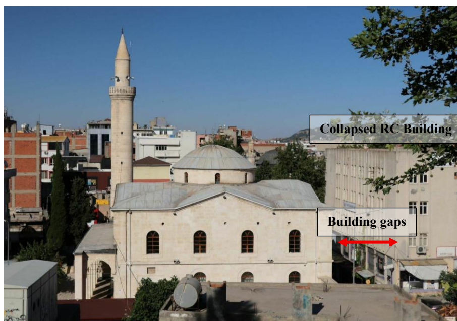
Figure 2-4 Adiyaman Grand Mosque and surrounding reinforced-concrete buildings before the 2023 Kahramanmaraş earthquakes, illustrating building gaps that exceed typical thresholds for pounding interaction. Source: Cultural Inventory (Ahmet Yurtbakan, Caner Cangül, Inan Kenan Olgar), kulturenvanteri.com
