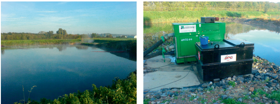
Figure 6.1 – Impression of the stabilization pond and pump for transporting the stabilized WWTP effluent to the UF-RO installation at the WWTP Sas van Gent
