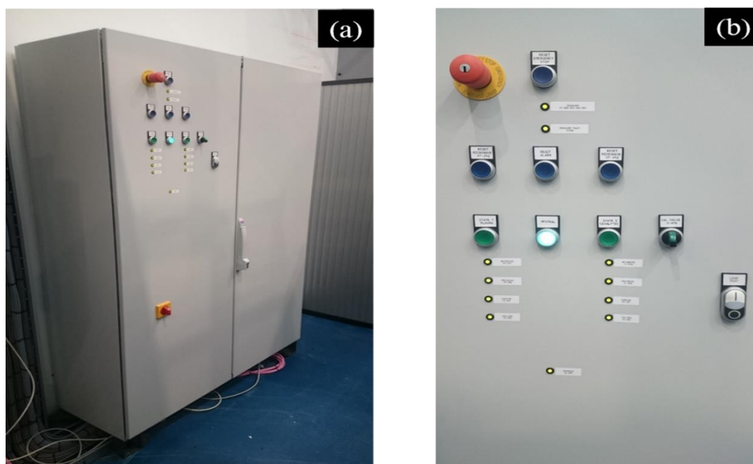
Figure 2.9 (a) cabinet of the control system and (b) manual buttons for reactor selection along with safety indicators
