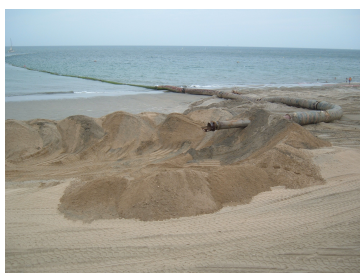
Figure 3.24: Beach nourishment device (Ehardt, 2007)
