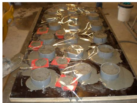
Figure 6-11: PVC pipes after filling with concrete
