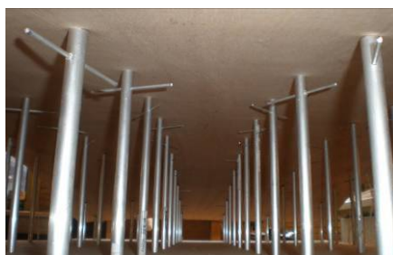
Figure 10-13: Bottom of the mould, middle supports
