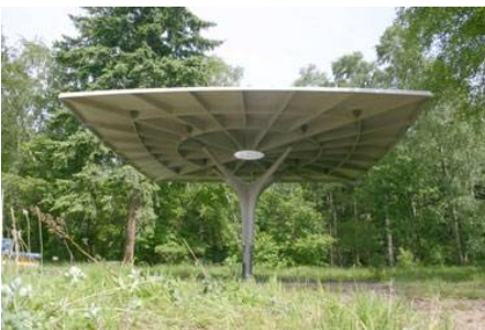
Figure 2-14: Canopy at sanatorium Zonnestraal [49]
