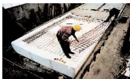
Figure 1-2: EPS formwork [1]
