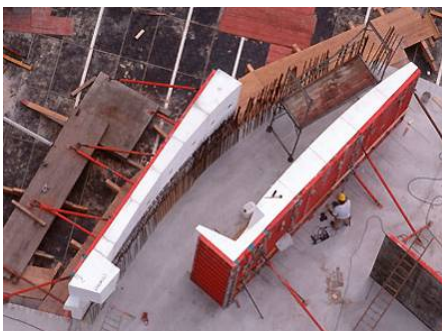
Figure 2-19: Foam formwork for Der Neue Zollhof [54]
