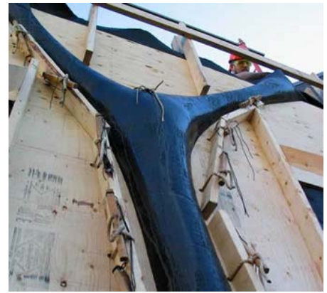
Figure 2-20: A fabric formwork for a column [54]
