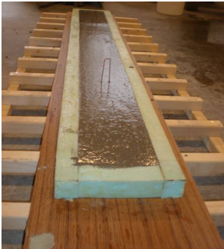
Figure 8-24: Mould filled with concrete
