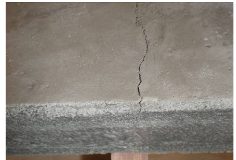
Figure 8-28: Crack, element out of the mould, top side
