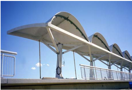
Figure 2-13: The Shawnessy LRT station [48]
