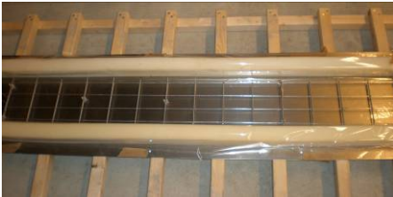
Figure 8-10: Steel plate formwork
