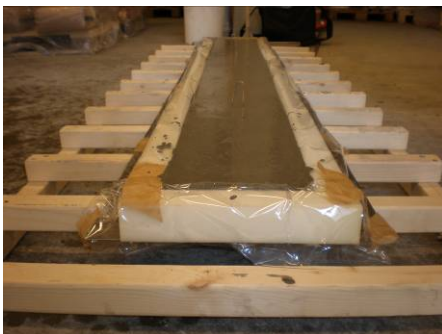
Figure 8-11: Formwork filled with concrete
