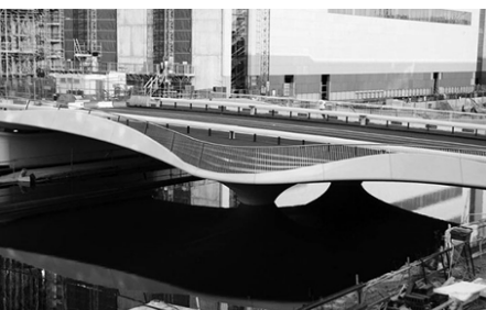
Figure 2-16: Spencer Dock Bridge [51]
