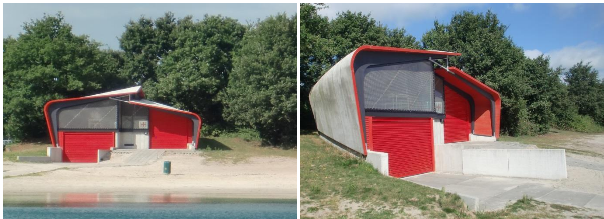
Figure 2.11 First aid emergency post in Galder, the Netherlands.
