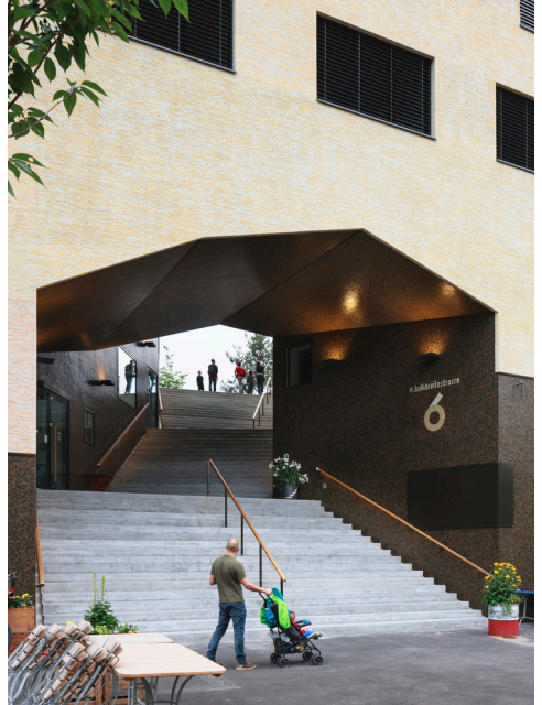
Fig. 13 Stairs to the courtyard ©Martin Stollenwerk (Source: Archdaily, 2018)
